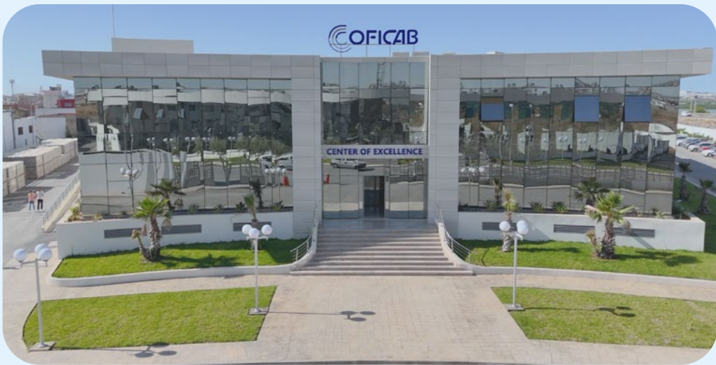
THE “NEW TUNISIA” PROJECT
