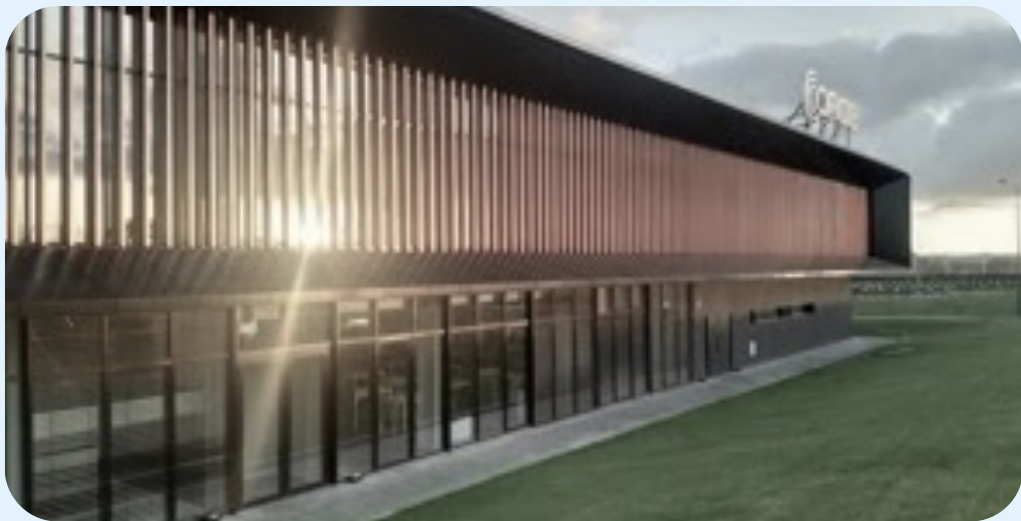
ECAD PROJECT, GUARDA
